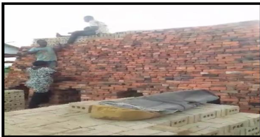
Fig. 6: Packing of dried bricks to form clamp kiln (Source: Fieldwork, 2023)
